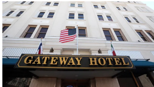
The Gateway Hotel at 104 S. Stanton St., in Downtown El Paso, is being renovated by owner Howard "Danny" Yun. He's reopened one floor with 25 rooms and hopes to have all 100 rooms open by the end of the year. RUDY GUTIERREZ/EL PASO TIMES
