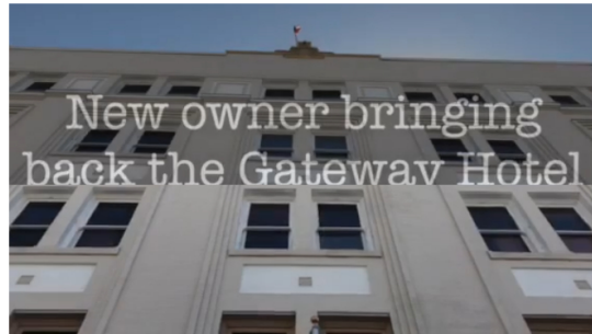
The Gateway Hotel downtown is coming back to life, fulfilling the dream of its new owner Rudy Gutierrez / El Paso Times
